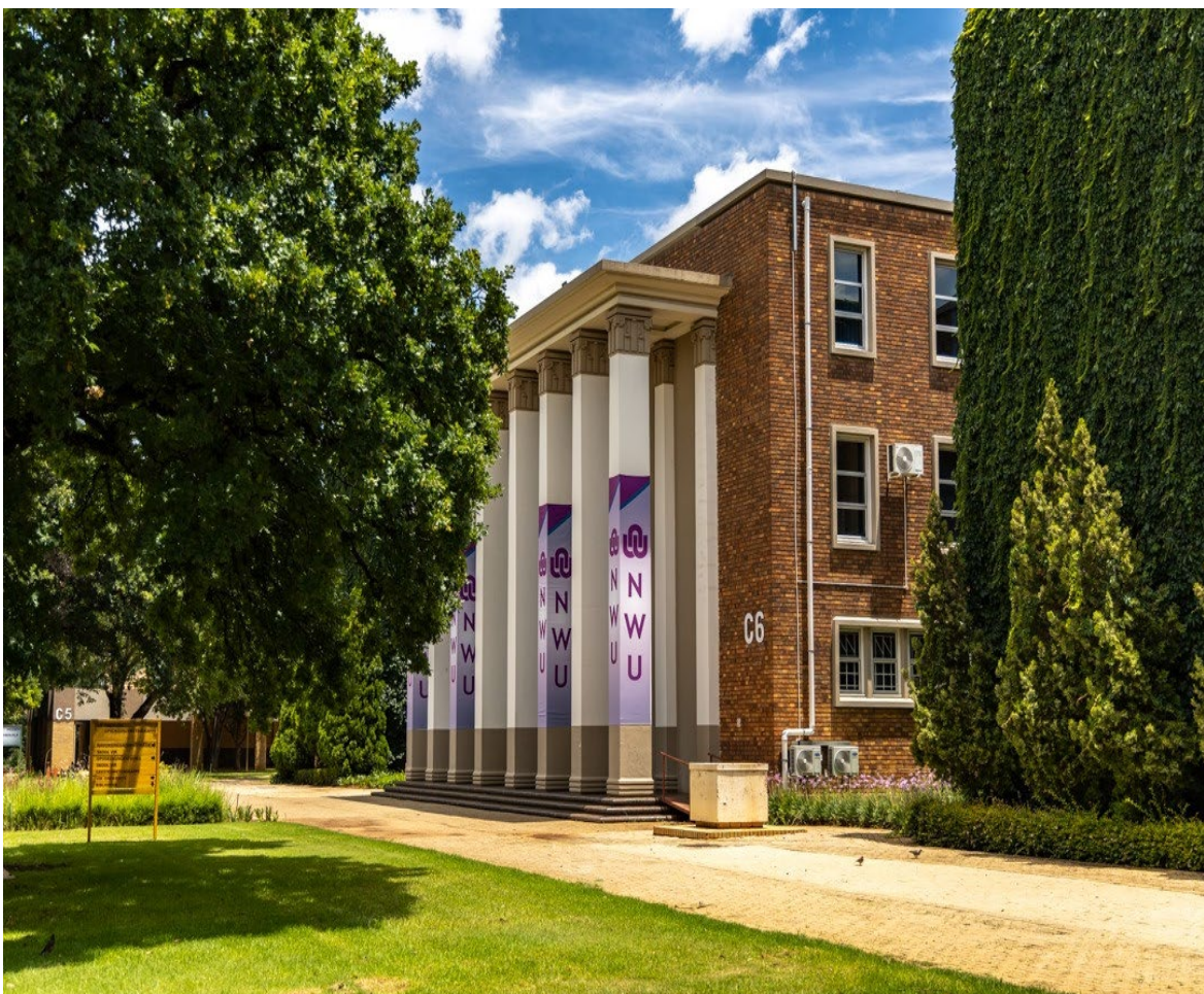
Figure 40: Building C6, Potchefstroom Campus
